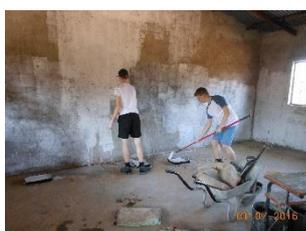
The work was hard. Lime-washing is difficult and soul destroying. It required a lot of motivation to keep the boys going. The PVA paint we put on top of the lime wash was also tricky. Malawians like to thin down their paint as much as they can which means that getting a good coating of paint on the walls requires quite a bit of
