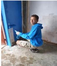
The blue gloss on the walls was a lot easier and went on in a satisfying way. The metal doors and windows were tough. The most paint that the builders had was the dark blue. We therefore thinned that down to use as undercoat. However, putting the gloss coat on top of a dark undercoat was very difficult – especially with the yellow top coat.
